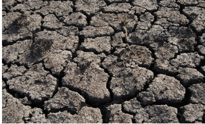
Fig. 1.1 Typical Cracks in Black Cotton Soil
