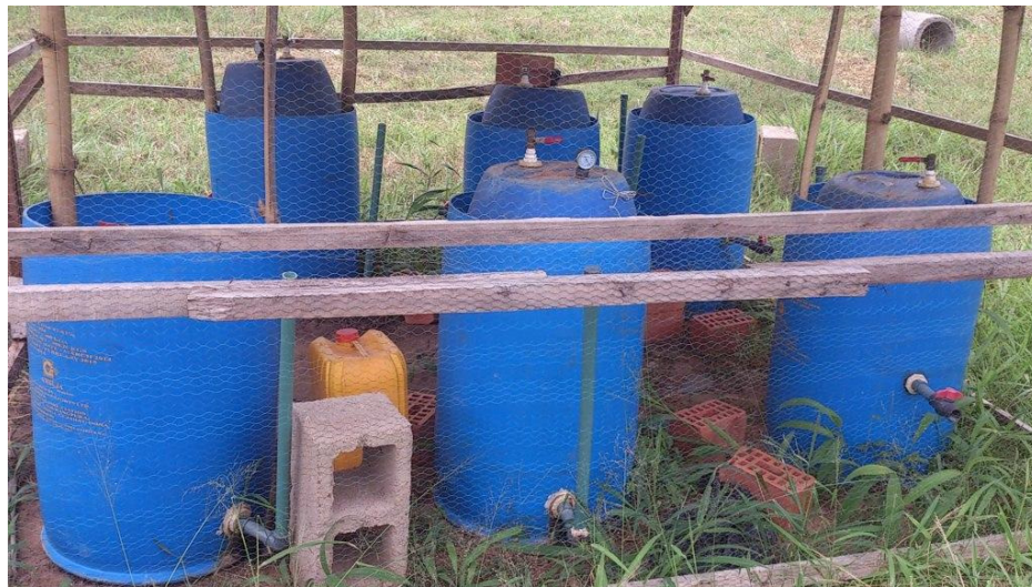
Figure 2: The five digesters under a shed.
