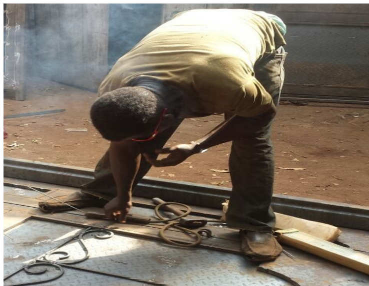
Plate 3: Welder at work
