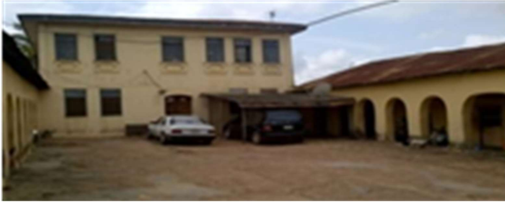
c) Patriarch & women section opening into the open fenced fore court (Islamic influence)
